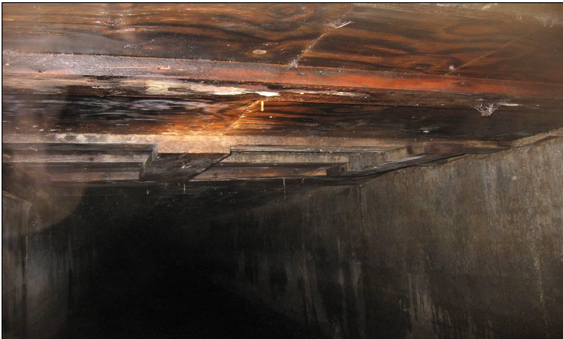
Figure 2.2 – Formwork in Wad Culvert at Seapoint Development on Clontarf Road
