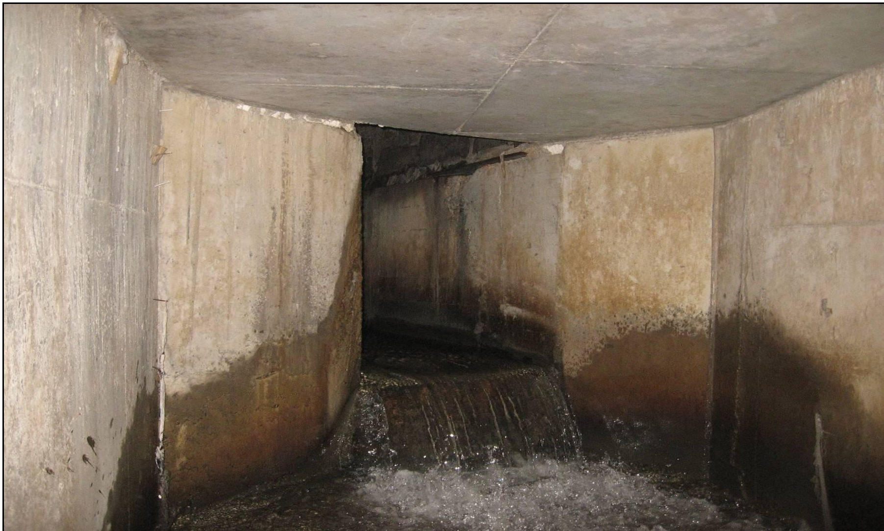
Figure 2.1 – Narrow section of Wad Culvert under Howth Road
